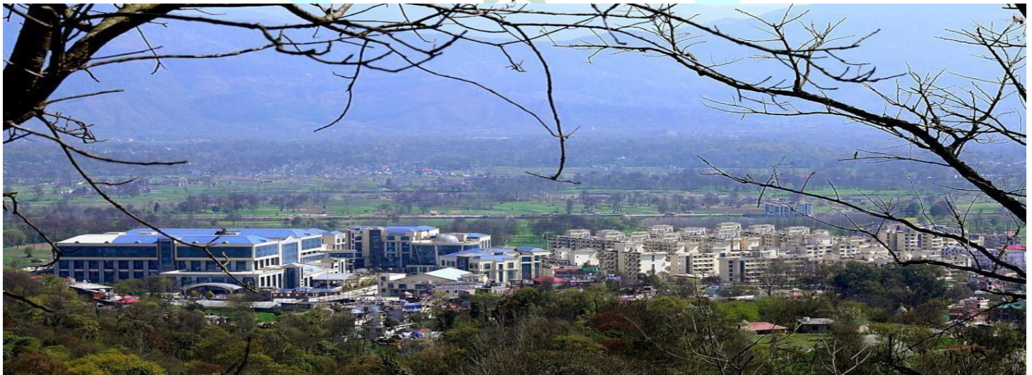
A VIEW OF SHRI LAL BAHADUR SHASTRI GOVT. MEDICAL COLLEGE & HOSPITAL, At NERCHOWK, DISTT. MANDI, HP
